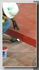
Holes from entrained air on the sides of the slab were filled with a mixture of Cabosil and the Ergon SC3300 to maintain the maximum chemical resistance throughout the production platform.
