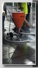
With our broadcast machine we applied a 1/2 lb. per sq. foot slip deterrent system of a graded #1 mesh throughout the 20,000 SF. This machine disburses the mesh evenly and without clumping for a more effective and uniform application.
